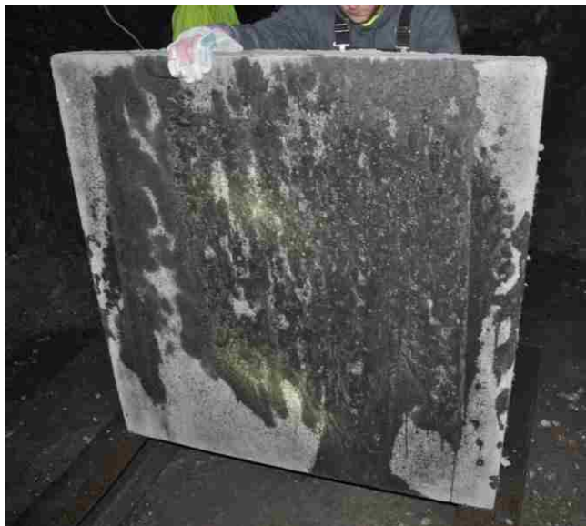
Figure 6.25. Bottom face of B-1-6F-3.5 after first detonation
