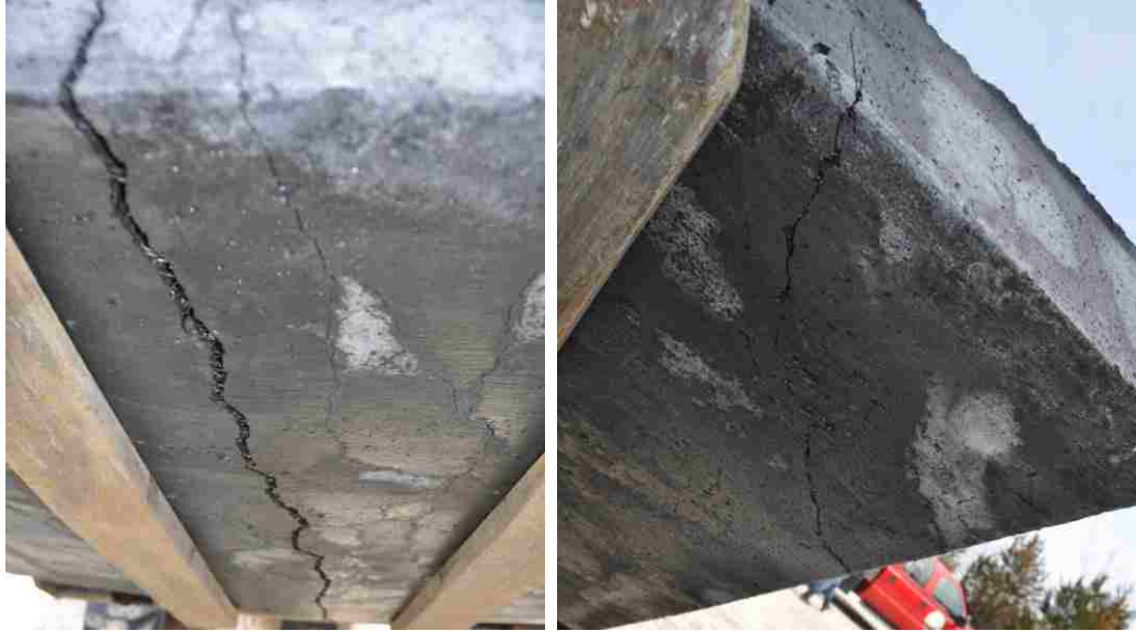
Figure 6.22. Panel B-3-2F-3.5 bottom face damage after both blast events
