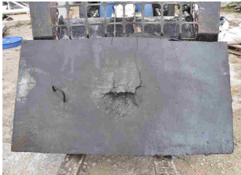
Figure 6.51. Spalling on tension face of H-3-6F-3.5 after detonation
